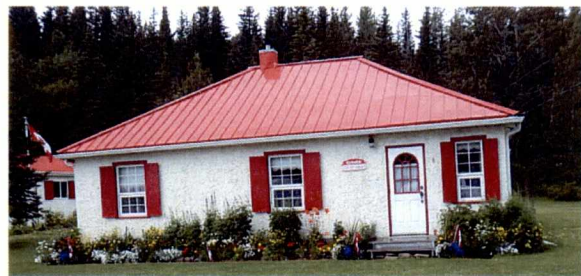
5. Existing Rustic Residential Dwelling
