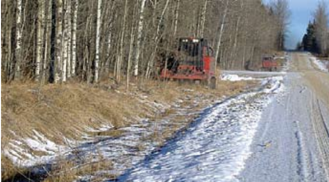
County crews clear the brush alongside roadways for weed control, to improve sightlines for drivers, and to reduce the risk of wildfire.
