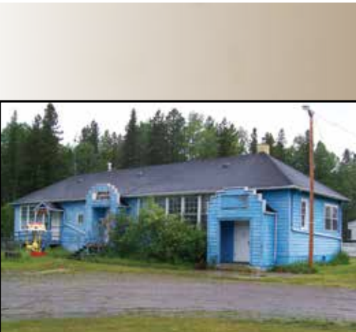
Bryan School is one of the many oneroom County School Houses that is receiving a commemorative plaque and is an example of one of the Yellowhead County schools that are no longer standing.
